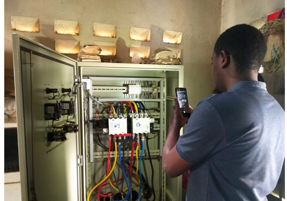
A CPHD team member installs the CT5 wireless monitor for the grid power supply in a hospital power house.
